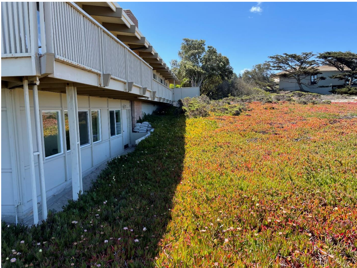
Figure 3: View along south side of existing house looking east.
