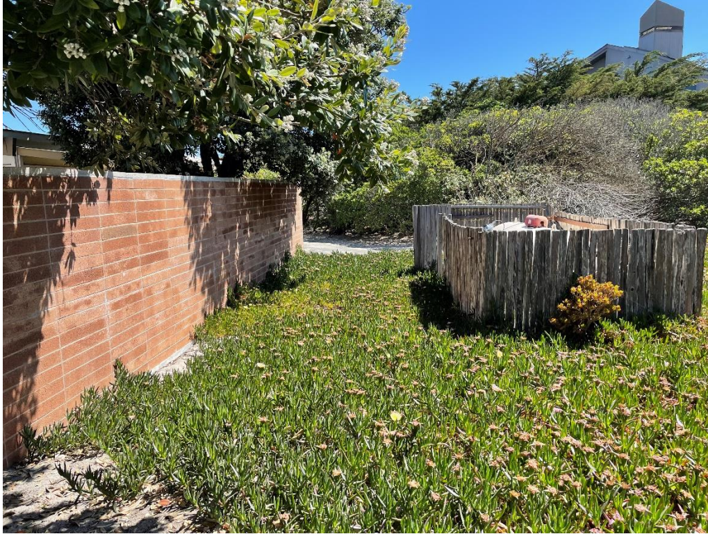
Figure 9: View along back (east) side of existing house at LP tank enclosure.
