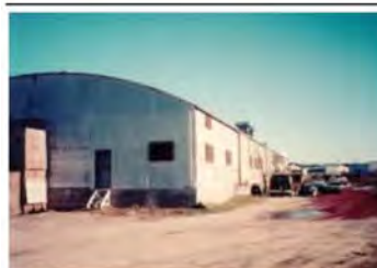
Numerous industrial facilities operate in Sand City
