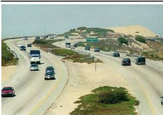
State Route 1 in Sand City
