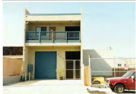
Housing atop an industrial building in Sand City
