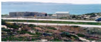
Pumping station on Bay Street
