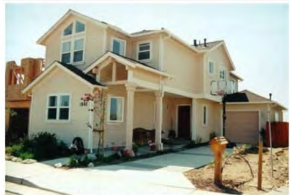
New housing in Sand City.
